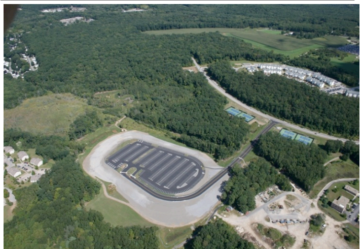
Remedial Work Plan Implementation UConn Landfill Closure
